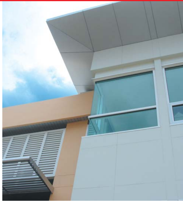
External Cladding Metro Park Condominiumtown, Bangkok
