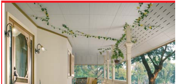
External terrace ceiling Using SCG SmartBOARD Wood Grain / Ventilated Wood Grain 4 mm. thick.
